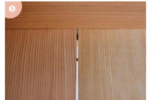
5 The bottom plate is reinforced with bamboo nails while leaving an appropriate gap.
